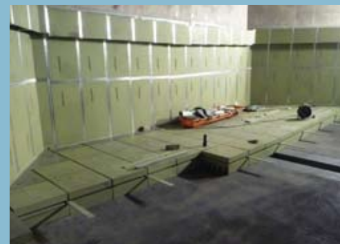
Installation der 578 Core-Catcher-Bodenelemente
