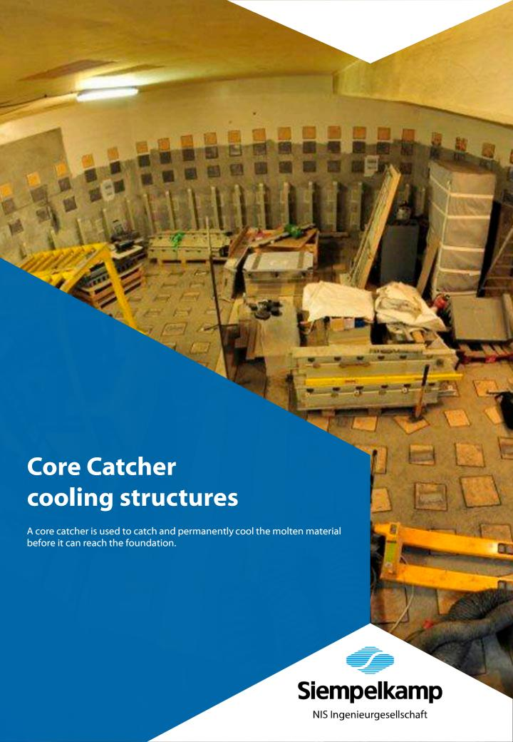
The Core Catcher is an essential part of the "Core Melt Stabilization System" in the EPR™ reactor and complements the primary safety systems of the EPR™ reactor, whose job is the reliable prevention, avoidance and control of nuclear accidents.
